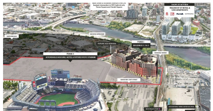
Phase 1 aerial: Citi Field in the foreground, Phase 1 buildings at right, and the Phase 2 stadium and housing area beyond.
