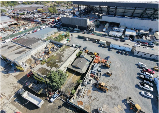
Closer drone view of the lot and existing structure, looking north toward the stadium site.
